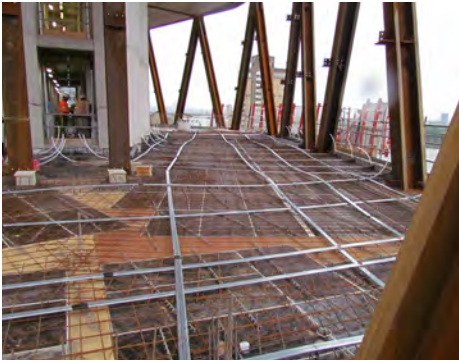
ABOVE High-strength tendons draped within a floor slab, waiting for the concrete to be poured at the Newfoundland tower, London
