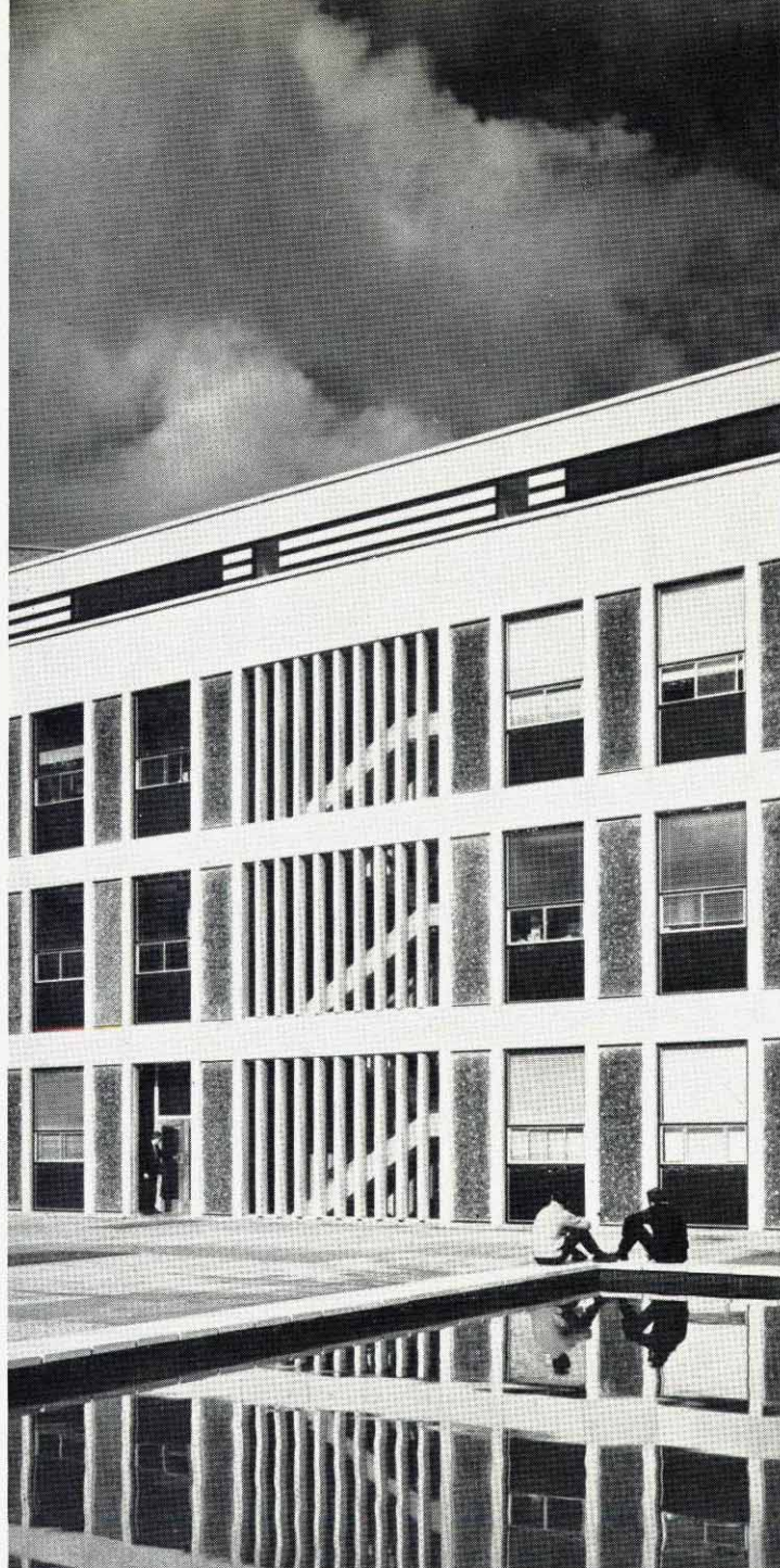
Above: View of a laboratory block, from the pool at upper deck level, showing a typical arrangement of cladding panels between pairs of columns, expressing the services arrangement within. Cavities behind the white horizontal cladding units at floor levels prevent streaking from rainwater.
