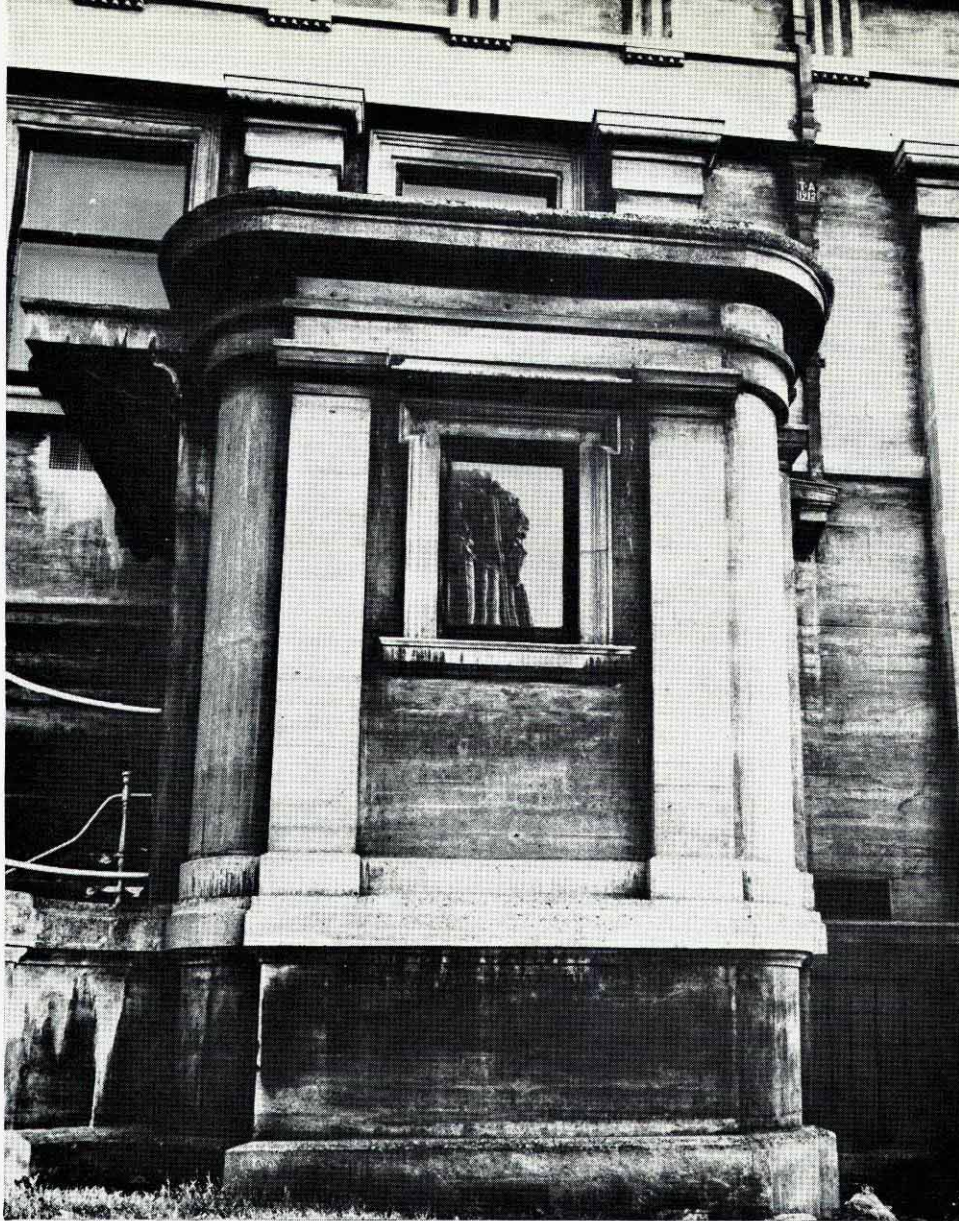
The entrance porch, built with astonishing precision of formwork. Note the use of horizontal and vertical boarding – the latter is 2\frac{1}{4} in. wide on the rounded corner pilasters.
