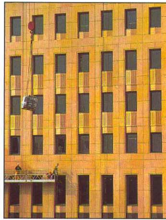
Storey-height panels on the Albert Embankment elevation
