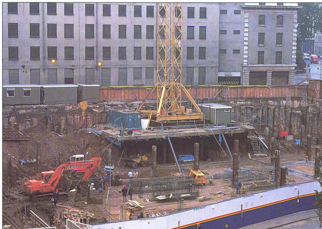
Advance construction of a section of ground floor provided a crane base
