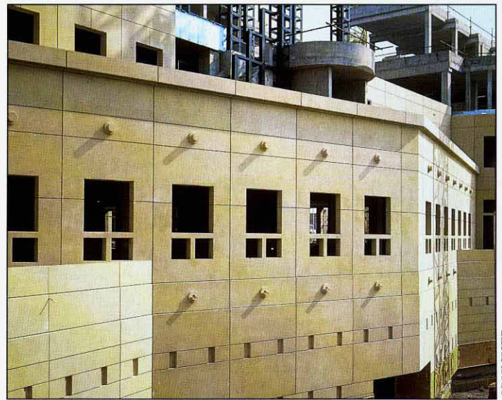
In some locations windows are drained through gargoyles
