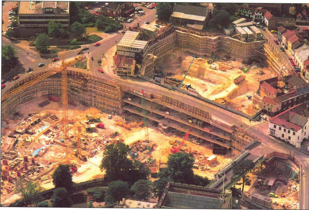
Early construction of the concrete road bridge saved nine months on the Castle Mall development, Norwich
