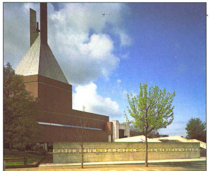
White board-marked concrete was extensively used
