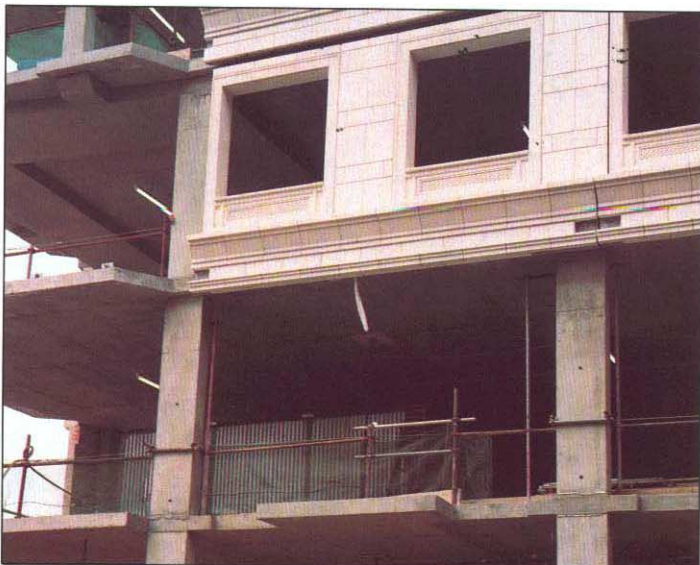
An in-situ frame with flat slabs matched steel for speed and saved £2/ft 2 (100 Ludgate Hill)
