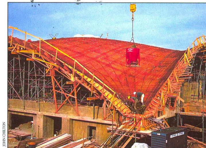
The four corners were concreted on the first day
