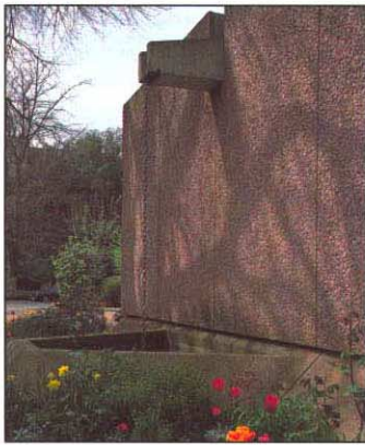
Water is drained from the ambulatory roof in a bold and interesting way
