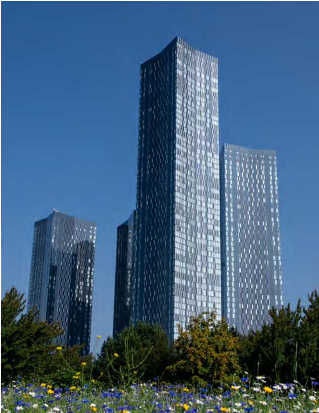
Left: Hanson's Regen GGBS cement was used on the four towers at Deansgate Square in Manchester. Mixes ranged from 40% GGBS in the main structural elements to 70% in the foundations and raft bases
