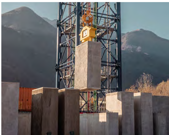
Above: As the jib lowers the blocks, the suspending cable drives dynamos to generate electricity. The blocks drop at about 3m/second and each generates around 1MW as it falls
