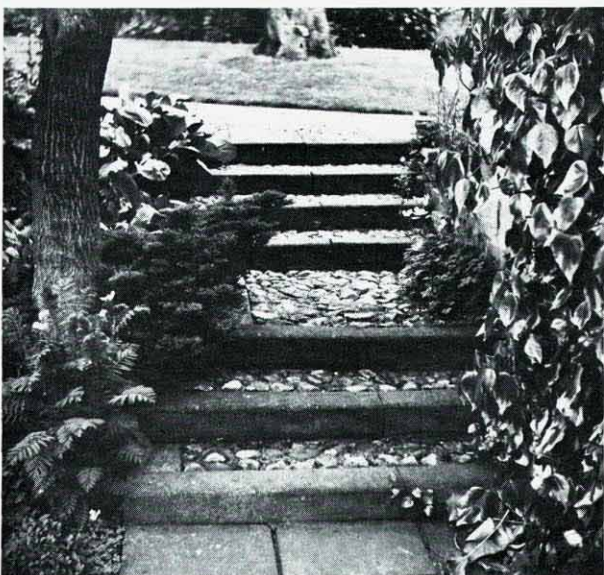
Above and below: Details of the paved terraces around the house showing the small precast concrete slabs infilled with cobbles or flints.
