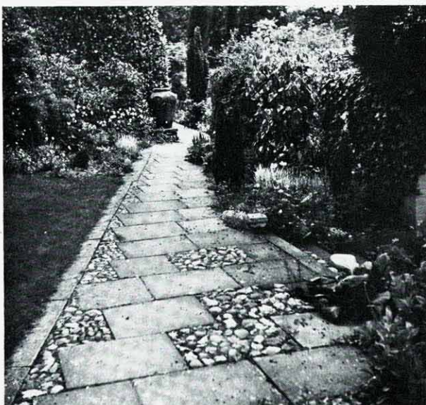
Above and below: Details of the paved terraces around the house showing the small precast concrete slabs infilled with cobbles or flints.
