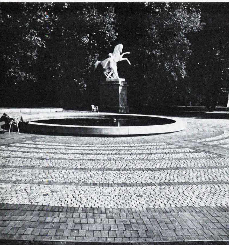
Concrete and granite paving slabs set in a circular pattern around a pool.
