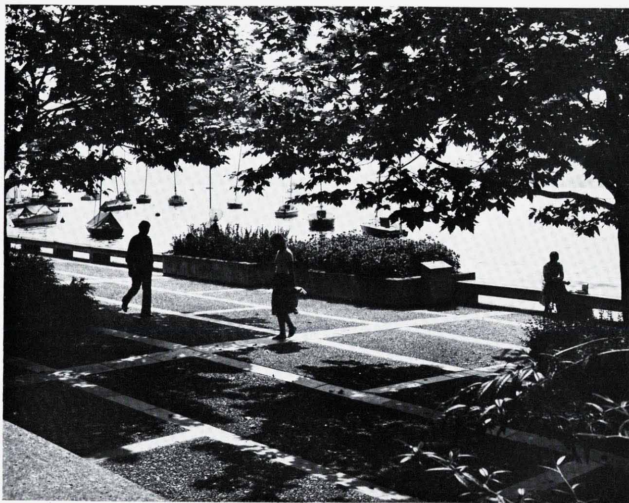
Excellent in situ concrete paving divided by precast slabs, Uto Quai – the promenade beside the Zürich-See.
