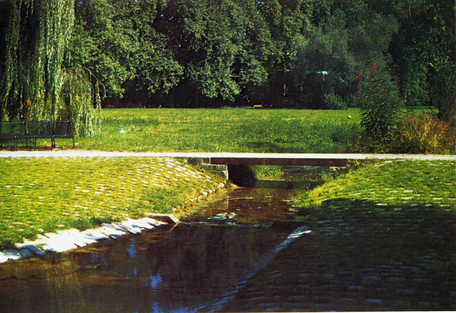
A footbridge formed of a simple slab crossing a stream, with grass and concrete paving on the banks.
