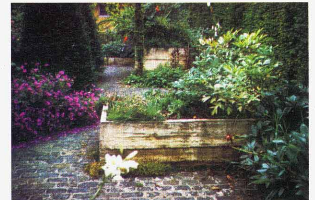
Upstand concrete border cast against railway sleepers to give character and texture.
