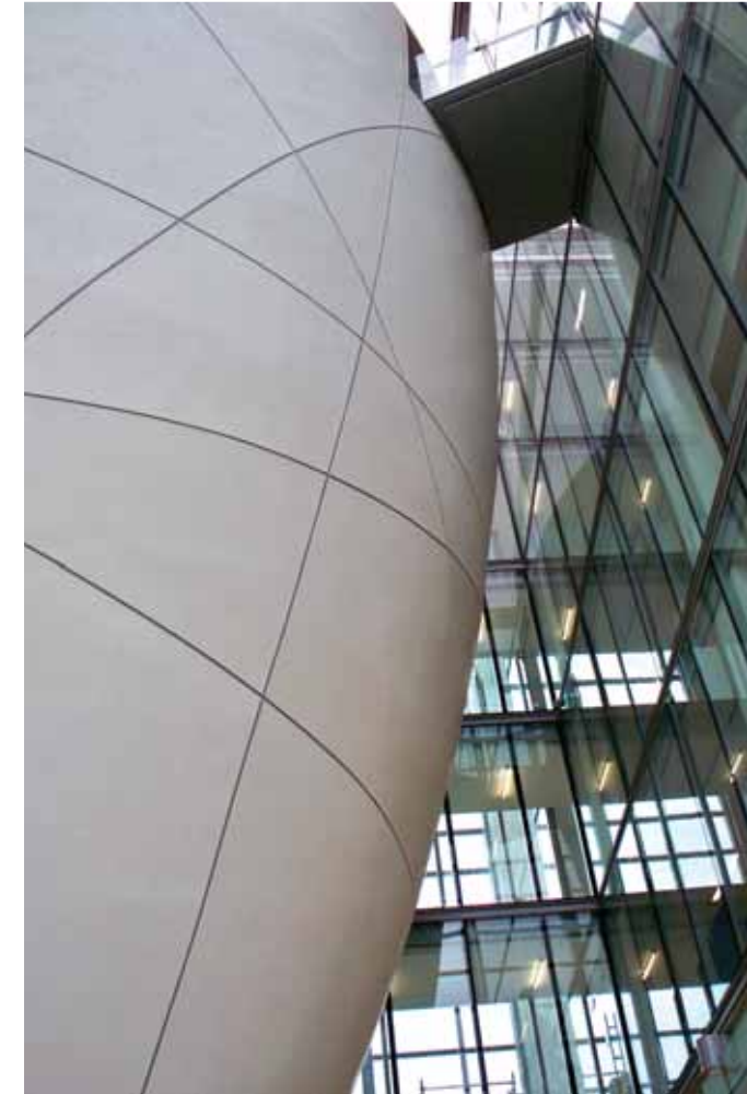
The Darwin Centre pod has a sprayed reinforced concrete shell.
