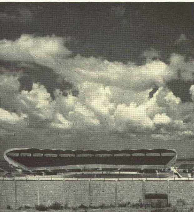
The stadium with its sweeping canopy of cantilevered shells.
