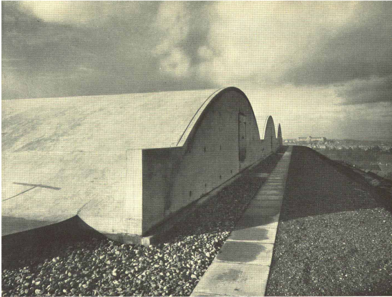
The concrete structure of shell roofs and end walls that encloses Humbleton High Reservoir. The irregular shape of this reservoir made necessary the flat-roofed portions at the ends.
