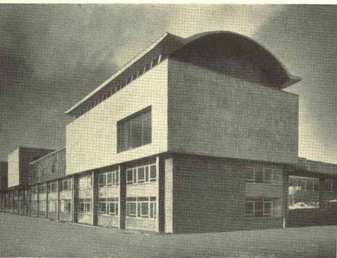
Above: The entrance hall block, with beyond, the south side of the factory, containing cloakrooms and offices. The entrance hall is faced with exposed-aggregate precast slabs in lightish grey. Below is brick; the gable end is ribbed in situ concrete. Below: The upper level of the boiler house, roofed with a steep shell of thin concrete.
