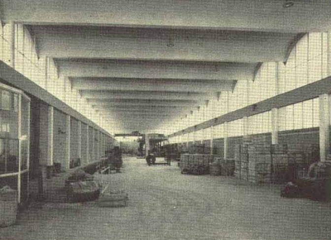
Above: The interior of the drug room, roofed with its twenty-six shells of concrete. Much light comes from glass spandrels in both sides and a continuous strip of glazing in the outer wall. Below: The mill room shells, seen from the roof of the main production area. The small down pipes, painted dull green, give an air of almost Victorian daintiness to this vista of narrow arches.
