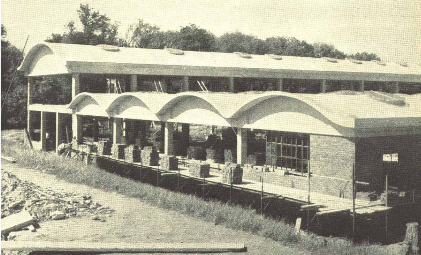
The maintenance buildings under construction. In the background is the main repair shop, in front the storeroom, with the general building on the right.
