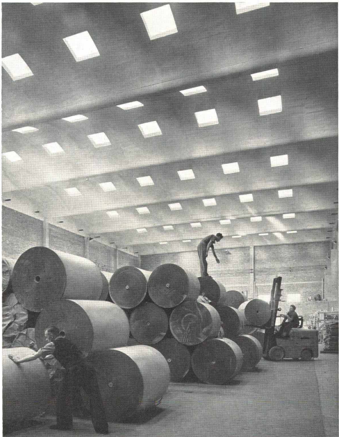
Interior of the reel store built across one end of the tuber machine room. This section of the building is roofed with symmetrical barrels pierced with square roof lights.
