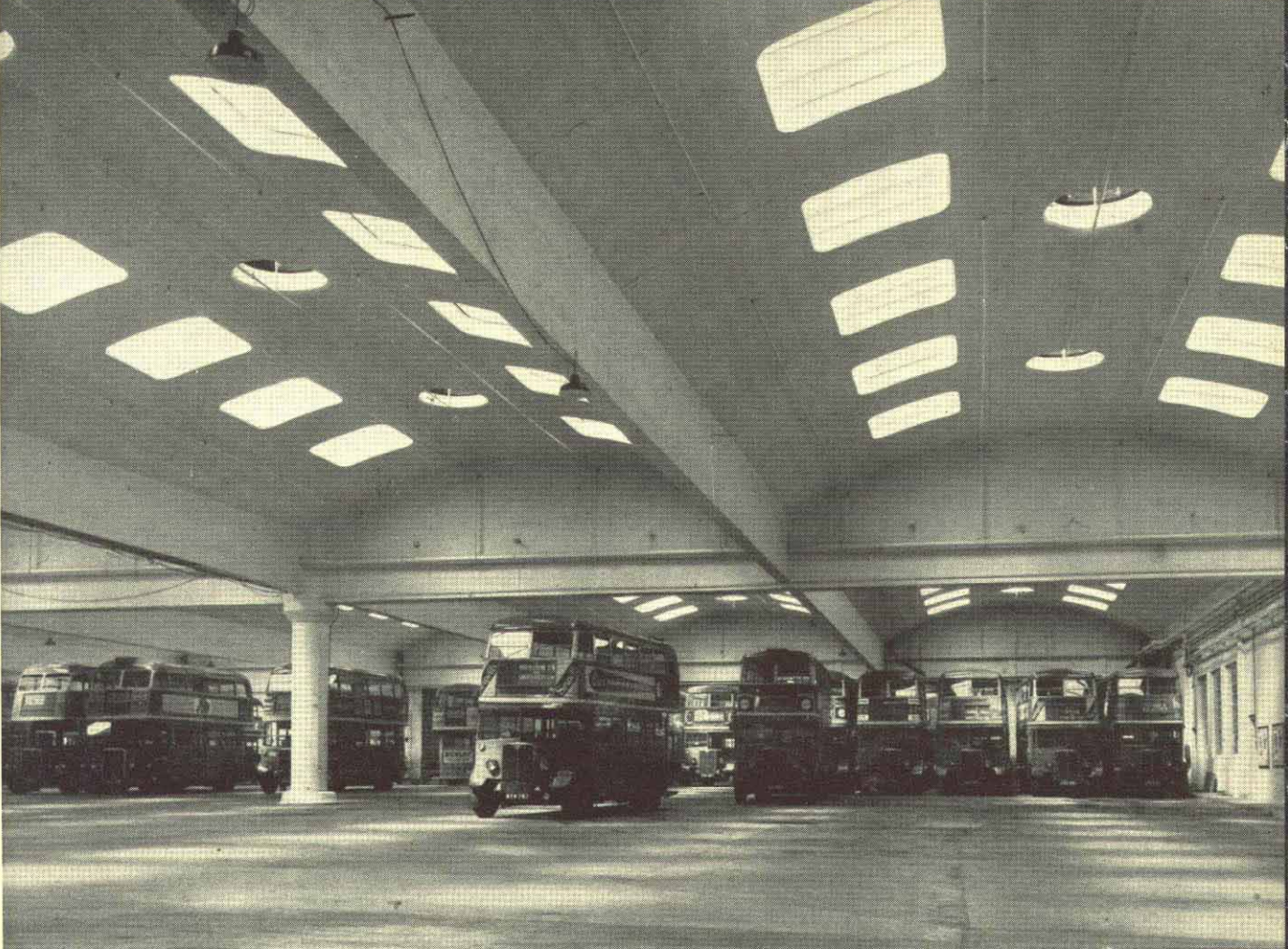
Part of the parking area at the new Bull Yard garage. Across the centre is the beam which carries both sets of shells and which is itself carried on two reinforced concrete columns, one of which is seen on the left.
