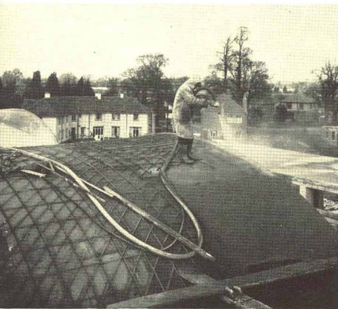
Placing the concrete of the roof by means of a pressure spray. It was later given a covering of bituminized felt.
