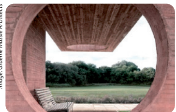
Pigmented board marked concrete Respite Pavillion, Scotland, by Graeme Massie Architects
