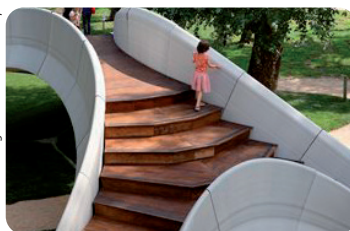
3d printed concrete Striatas bridge, Venice, by Zaha Hadid and Block Research Group
