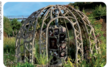
Fabric Formwork The Root Dome at The Eden Project, Cornwall, by Concept Shed Ltd
