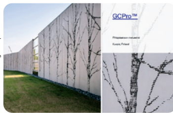
Surface retardant treated concrete Pihlajalaako sound barrier, Finland, by Ramboll and Graphic Concrete
