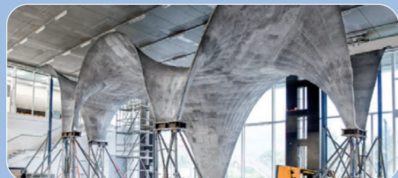
Ultra thin shell concrete structure Hilo, Munich, by supermanoeuvre and Block Research Group
