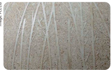
Acid-etched concrete Bromley South Station, London, by TBA
