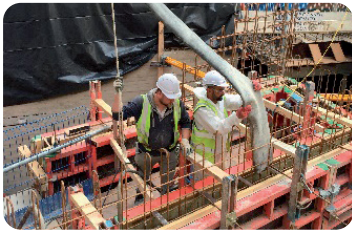
In-situ concrete The Royal College of Pathologists, London, by Bennetts Associates
