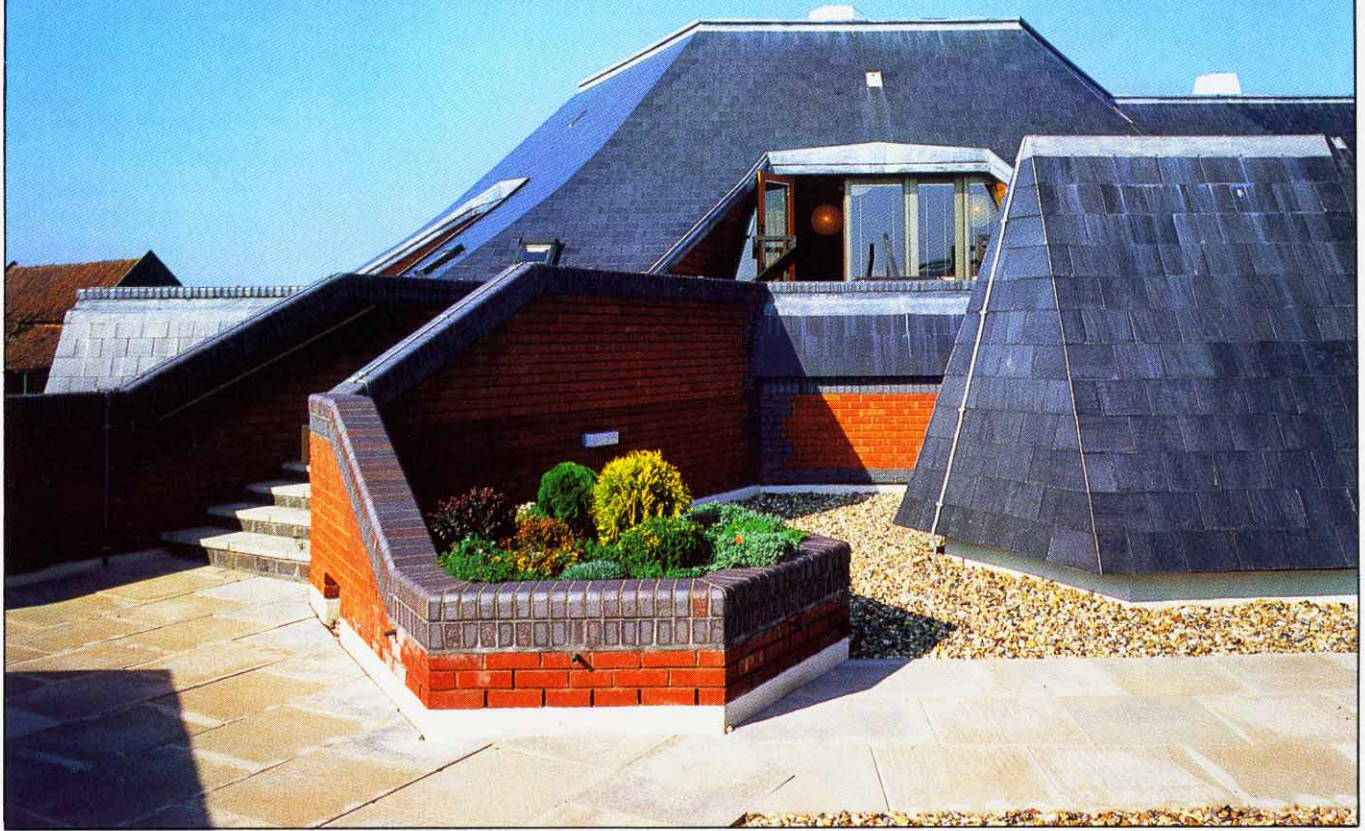
Concrete-paved rooftop terrace and asbestos-cement slate roof covering. (Photo: Architects' Journal)
