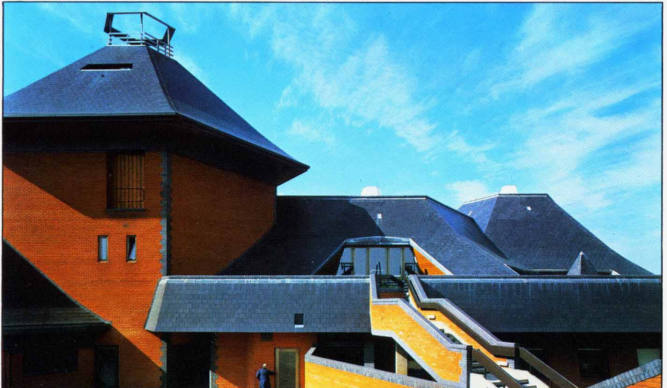
Close-up of the exterior showing the importance of the roofscape, seen here covered with asbestos-cement slates. (Photo: Architects' Journal)
