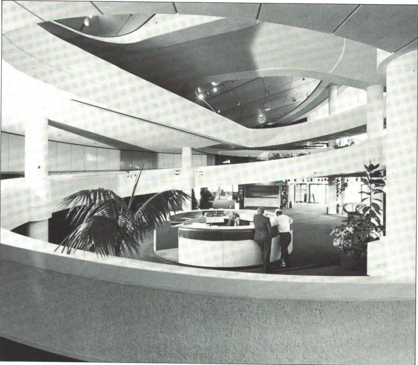
Below: The design of the ramp is based on sweeping curves and executed in high-quality white concrete.
