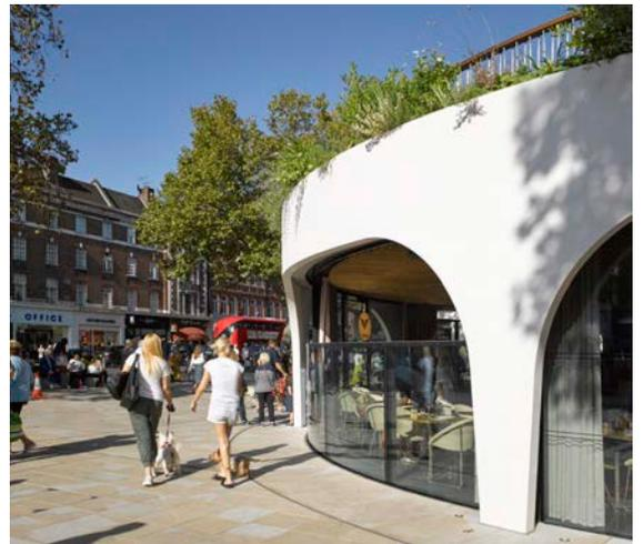
We chose a white concrete, with an off-white fine aggregate of quartz and a coarse aggregate of dolomite. The front and back surfaces have been acid-etched to give a slight lustre to the quartz – with curved concrete, you really want to do as little finishing as possible. But within the arches, we heavily ground and polished the reveals to show the pale-grey and blue dolomite stones. Conceptually, it reinforces the idea of a continuous ribbon being cut to form these openings.
