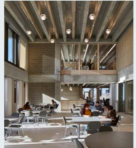
double-T structure. Closer examination reveals that the aluminium-framed woodwool slabs also carry features such as lights and smoke detectors.
