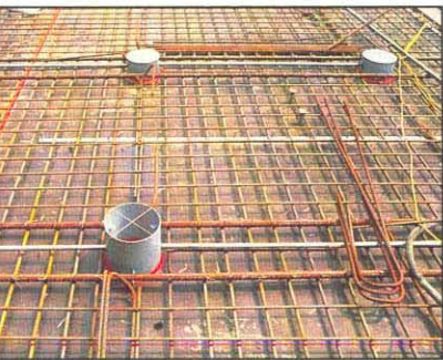
Cast-in light fittings supported the reinforcement
