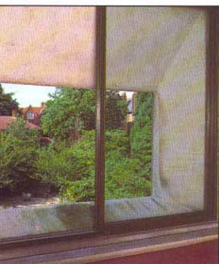
Dull surface of inner face of a hooded window surround disfigured by uncontrolled water
