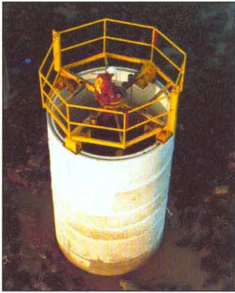
Fixing reinforcement from the working platform
