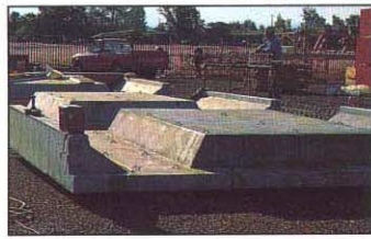
Concrete forms were used to cast the 40 segments
