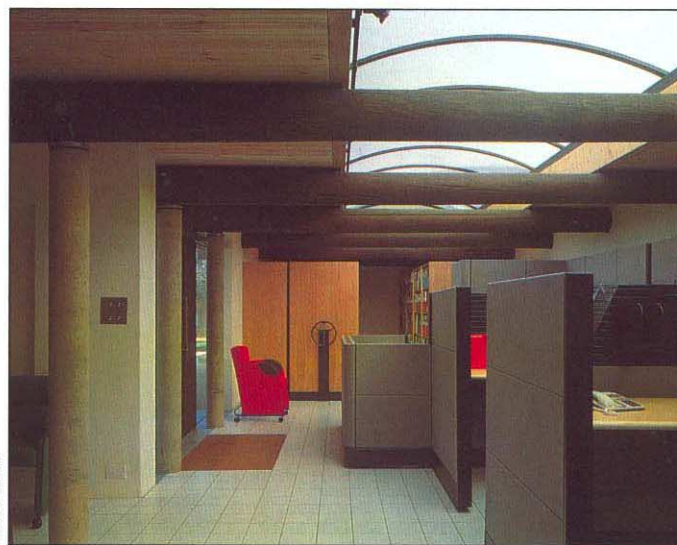
Where glazing replaces solid walls, the roof is supported on circular concrete columns
