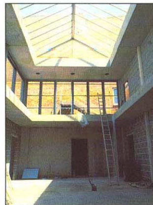
The thermal mass of the structure damps out temperature extremes
