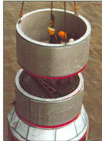
A precast ring is lowered onto the epoxy joint
