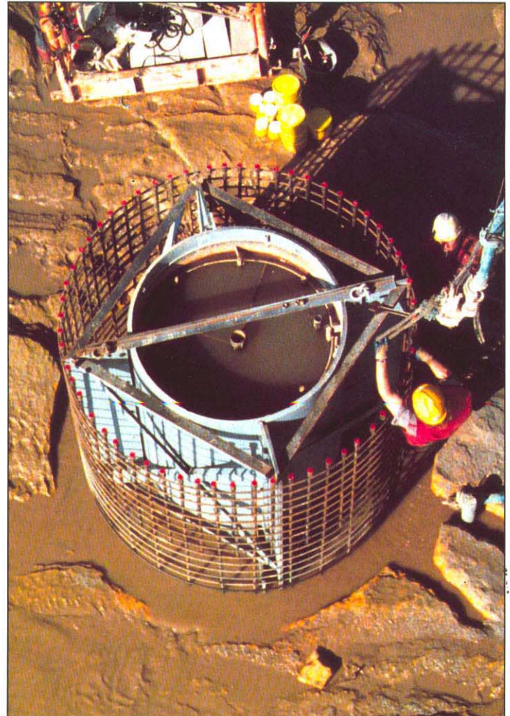
Pile-cap reinforcement fitted to the pile at low water
