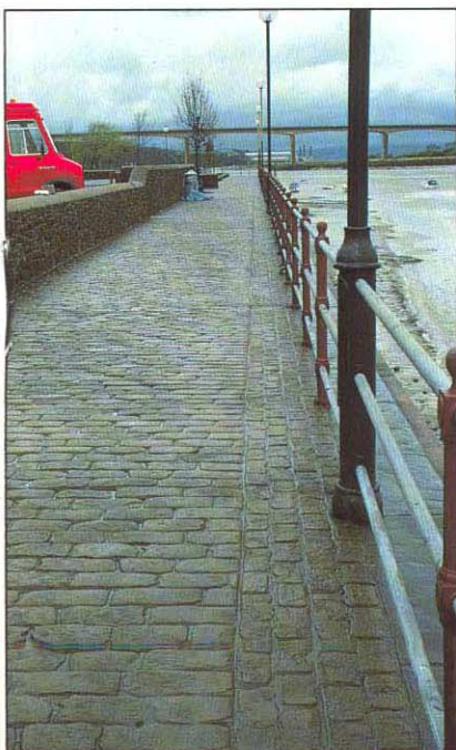
In-situ concrete with the appearance of traditional paving
