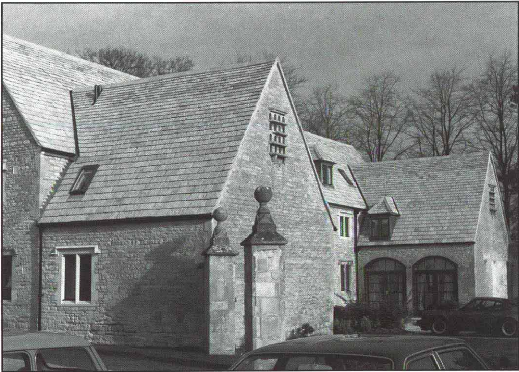
Below: Two views of the refurbished stable block at the Weston Manor Hotel which has new Bradstone precast 'Cotswold' slates on the roofs – visually and economically an acceptable alternative to replacing the roof with new stone slates.
