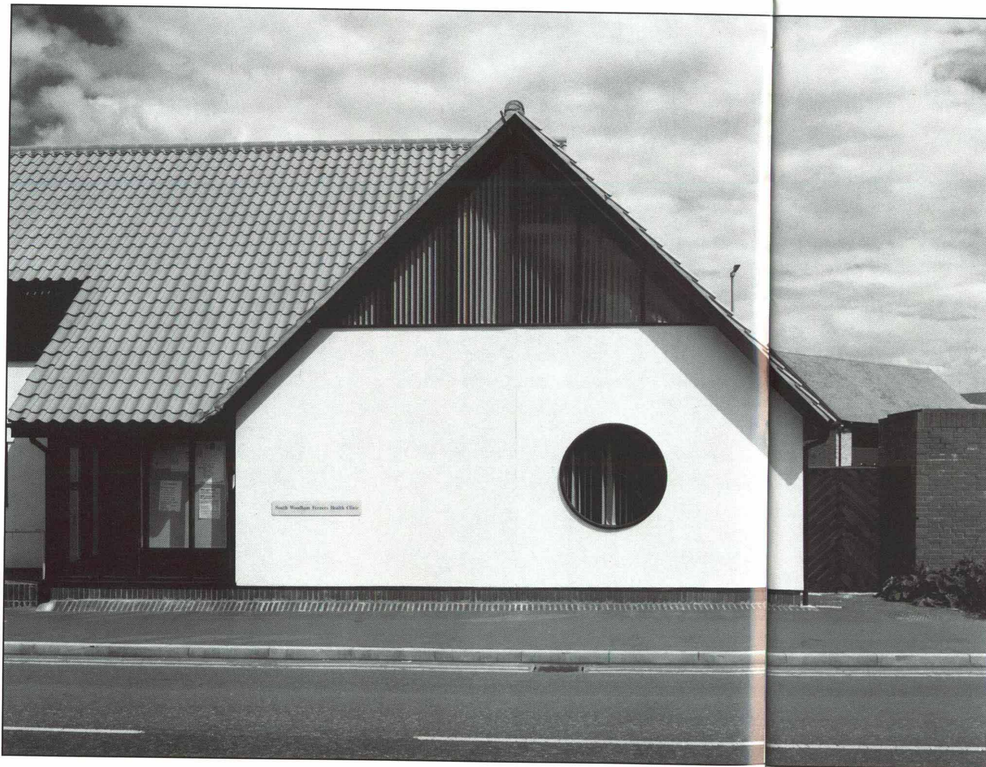
Left: Gable detail of the Health Clinic. Walls are of rendered aerated concrete blocks.
