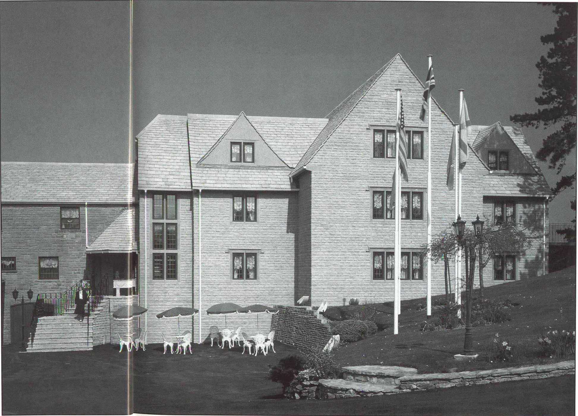
Below: General view of the new extension to the Hatton Court Hotel at Upton St. Leonards which has walls of Bradstone precast masonry blocks in the new Squared and Pitched Walling range and in a weathered Cotswold colour to complement the original building. The pitched roofs are clad with Bradstone 'Cotswold' roofing slates in a Weathered Buff shade.
