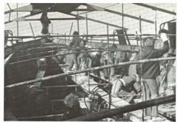
Planners working on the ferro-cement hull
