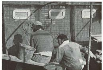
Planners applying mortar to the layers of galvanized mesh in the 1 1/16 in thick ferro-cement hull.
