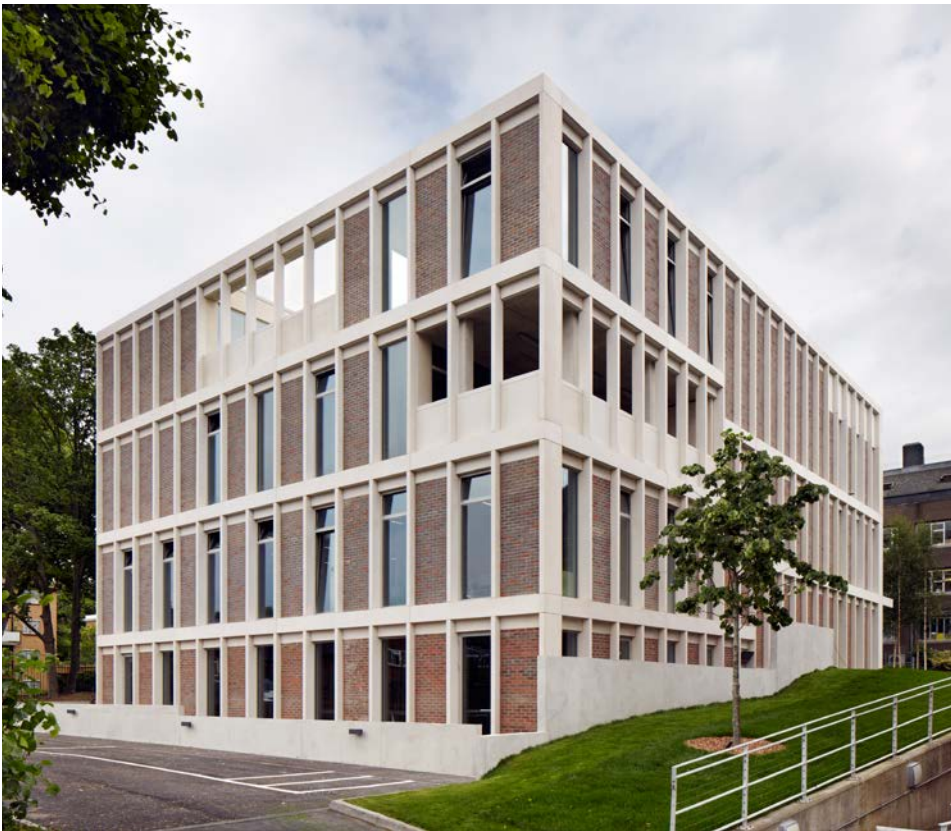
ABOVE The concrete frame of Duggan Morris Architects’ Ortus learning centre in south-east London contains 50% GGBS. Watch a Concrete Elegance presentation by the architect at www.concretecentre.com
