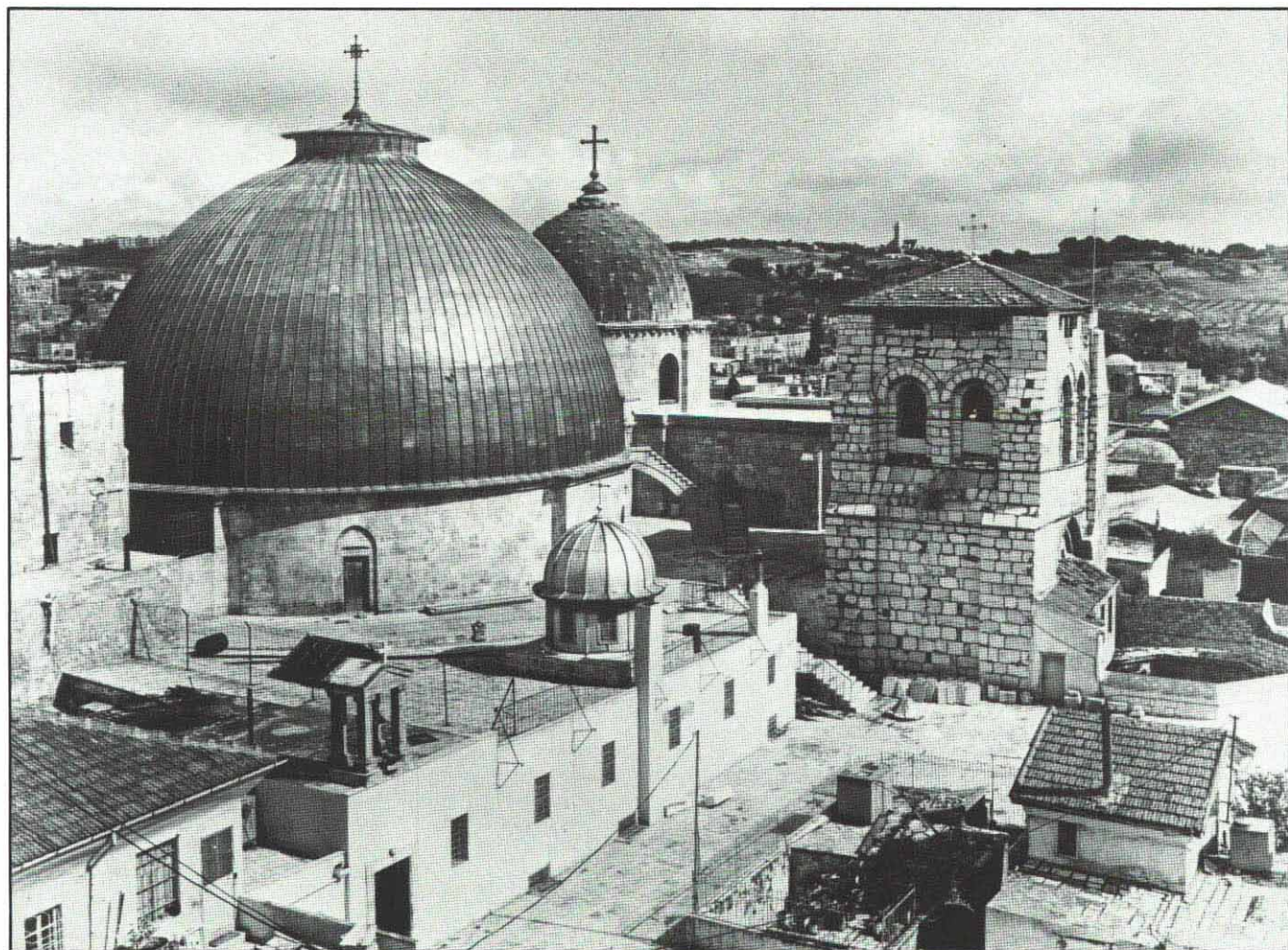
The restored dome in the foreground with its new lead-covered concrete shell.
