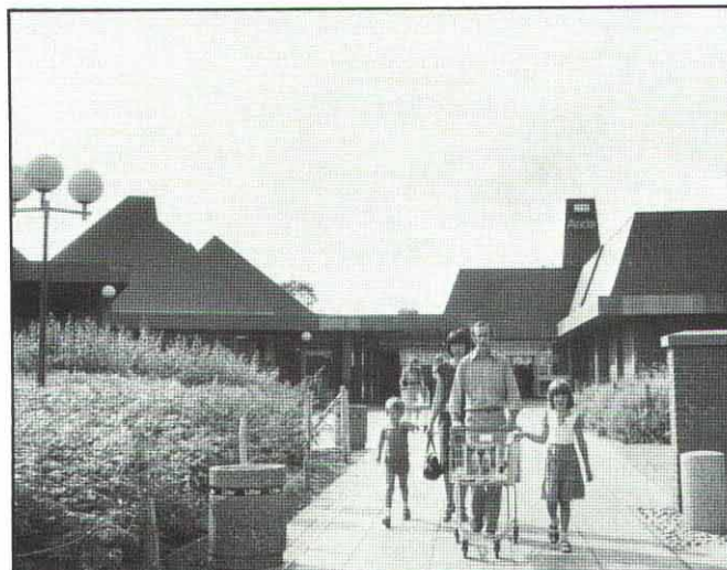
Top right: The steeply pitched roofs are covered with asbestos-cement slates.
