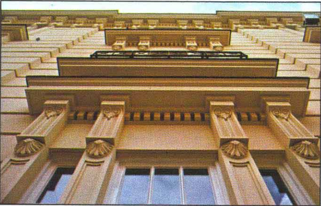
The restored Queen Street facade. Sills, mullions, window heads, cornices and mouldings are of precast concrete. Infill areas between are of rendered brickwork. All surfaces have been painted a matching cream. (Photo: Ormonde Photographics).
