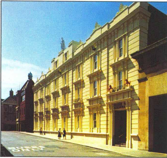
The restored Queen Street facade. Sills, mullions, window heads, cornices and mouldings are of precast concrete. Infill areas between are of rendered brickwork. All surfaces have been painted a matching cream. (Photo: Ormonde Photographics).
