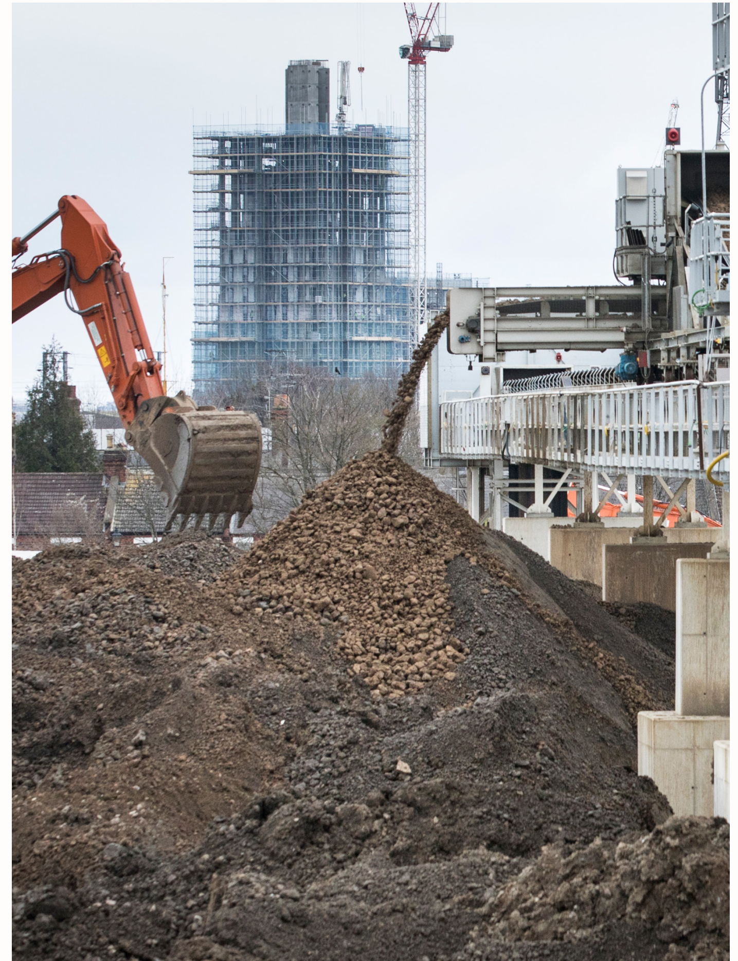
Extraction of site-won London Clay | Ex-Clay project
