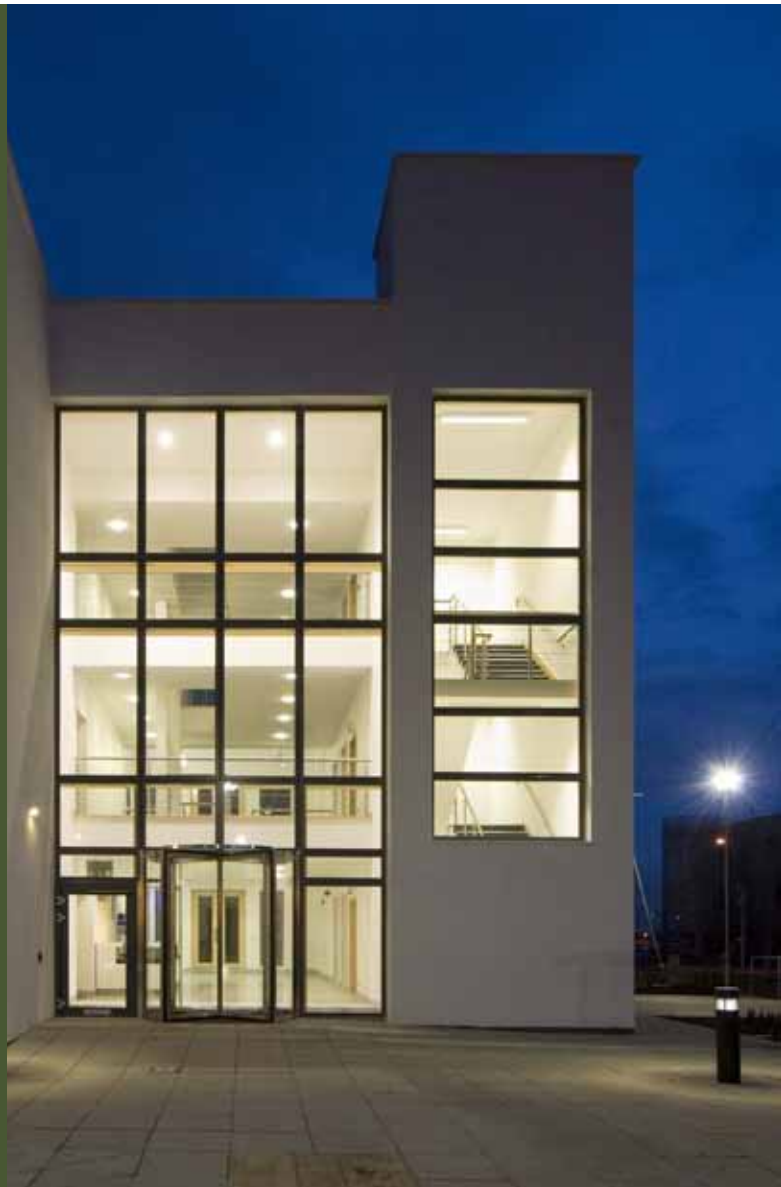
Innovate Office, Leeds utilises the thermal mass of concrete as part of an energy efficiency strategy that has been rewarded with a BREEAM Excellent rating.
