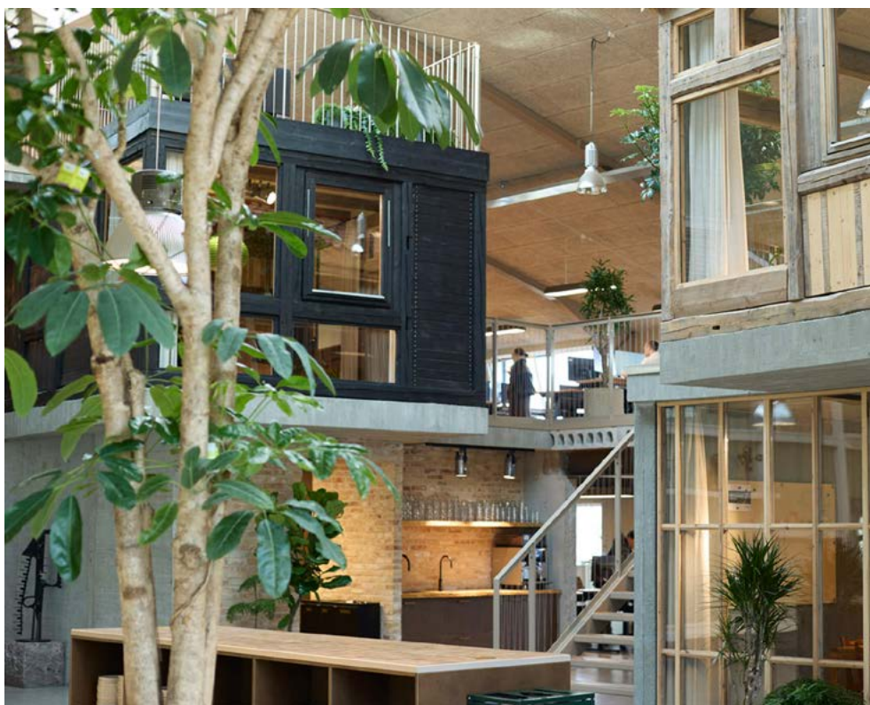
Left: Just outside Copenhagen, 3XN and GXN designed a headquarters for demolition company Tscherning, using almost solely reclaimed materials from its projects. In collaboration with the structural engineer, Tscherning tested different extraction methods and reused hollowcore slabs as “new” walls and floors
