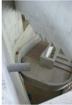
Precast formwork for Experian Data Centre Sheppard Robson
