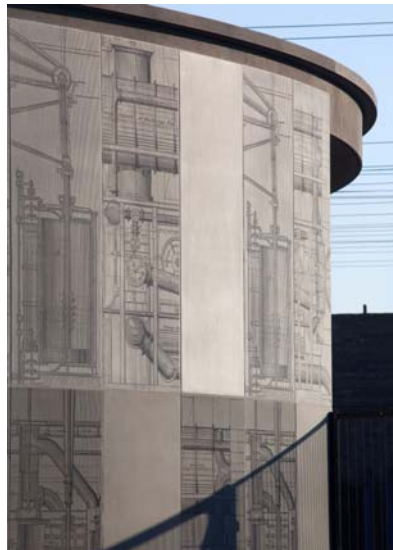
Pudding Mill Lane Pumping Station John Lyall Architects
