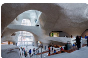
Sprayed concrete Richard Gilder Center, New York, by Studio Gang
