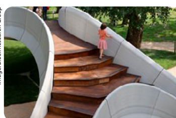
3d printed concrete Striatum bridge, Venice, by Zaha Hadid and Block Research Group
