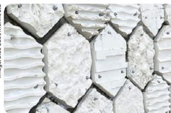
Textured concrete Mumbles Sea Hive, Wales, by Blue Cube Marine Ltd, using Reckli rubber form liners
