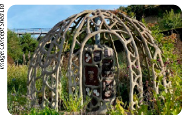
Fabric Formwork The Root Dome at The Eden Project, Cornwall, by Concept Shed Ltd
