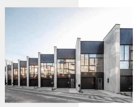
abandoned buildings in North Jutland. And the aggregate for the concrete, which is used everywhere from the foundations to the floor slabs to the roof, is 100% recycled from the surrounding area.
