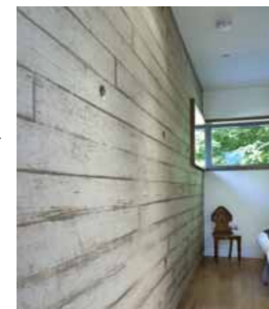
Opposite A concrete spine wall runs through the property linking the two buildings. Top Glazed doors to the living area retract to open up the house. Above One of the ground-floor bedrooms. Left Acrylic-treated shuttering achieved the best concrete colour and timber relief.
