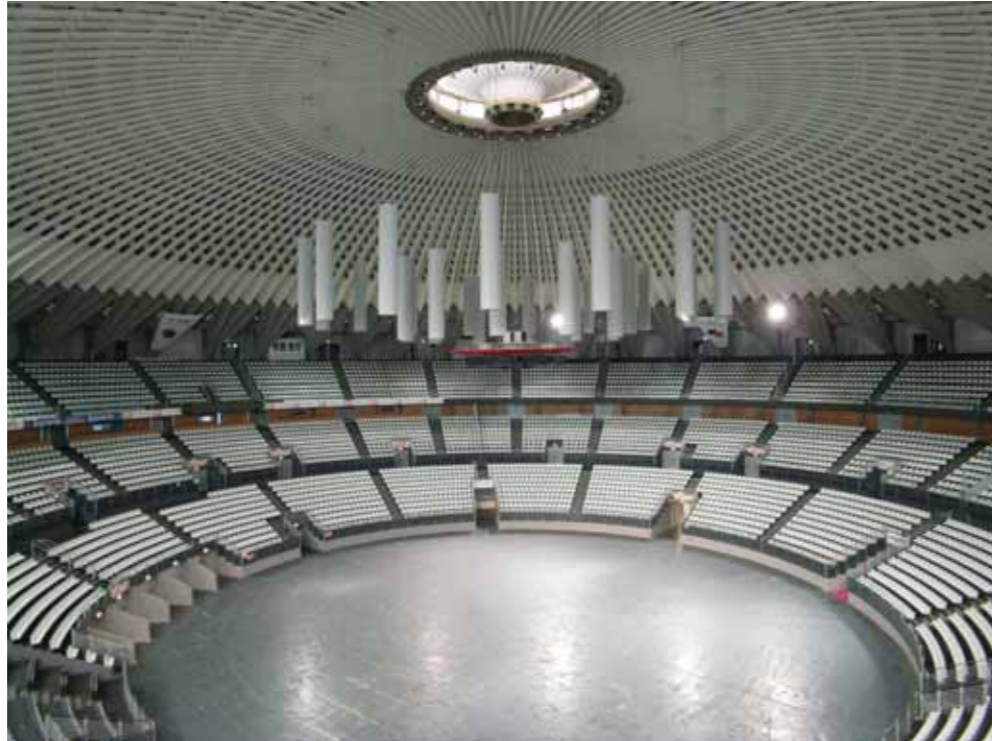
Above The Palaeur has been adapted by owner All Events with the addition of an acoustic system at the intrados of the dome and politically neutral white seats.
