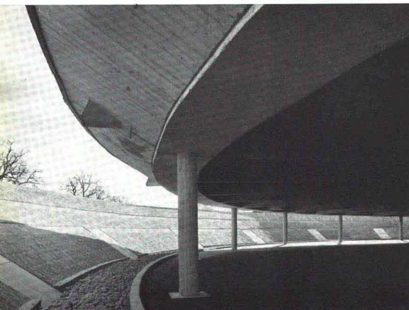
Left, above: The massive triangular-section ring beam at first-floor level carries core and peripheral loads down to 14-in. slab columns.
