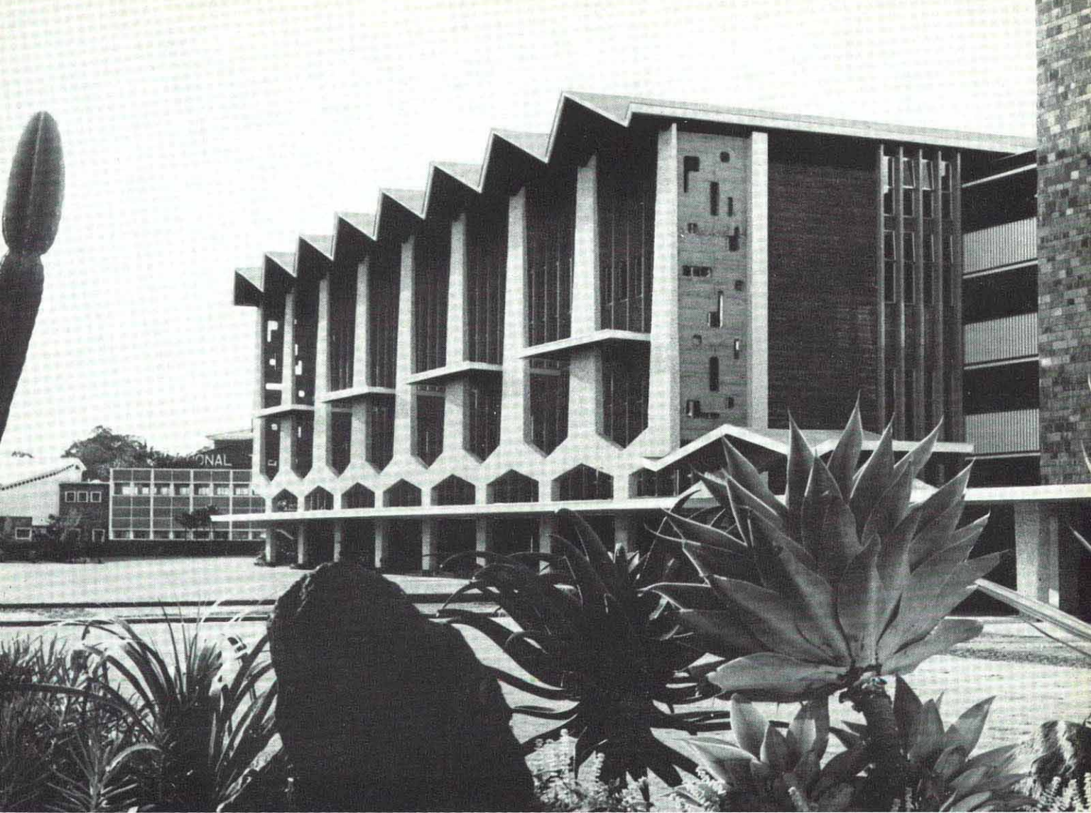
The façade of the library block, showing the folded plate roof, and the vertical and horizontal brises-soleil.
