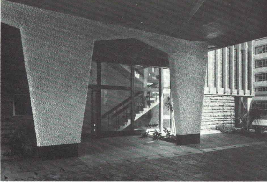
Below the entrance canopy; the supporting piers are faced with large Kenya marble aggregate. Paving textures have been given particular attention.
