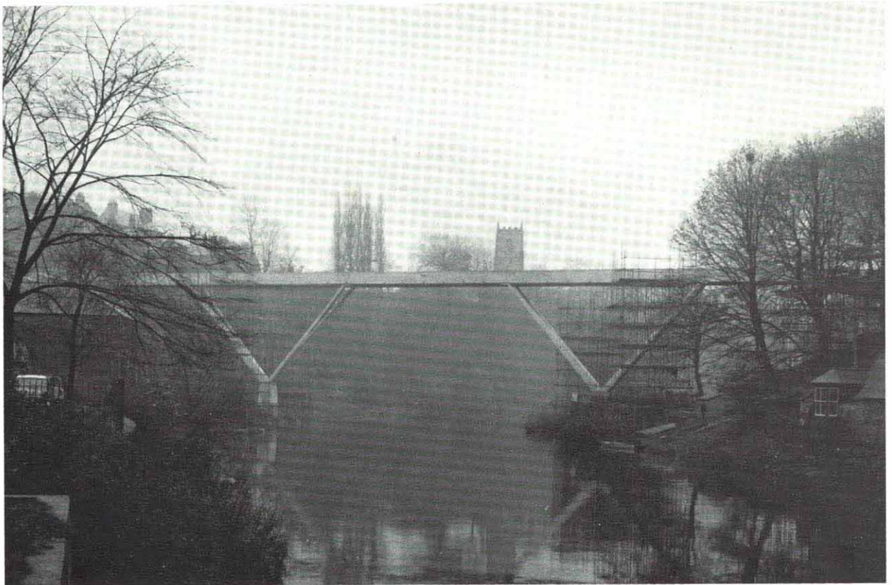
Misty weather in the Wear valley blurs the outlines of the new bridge among the trees.
