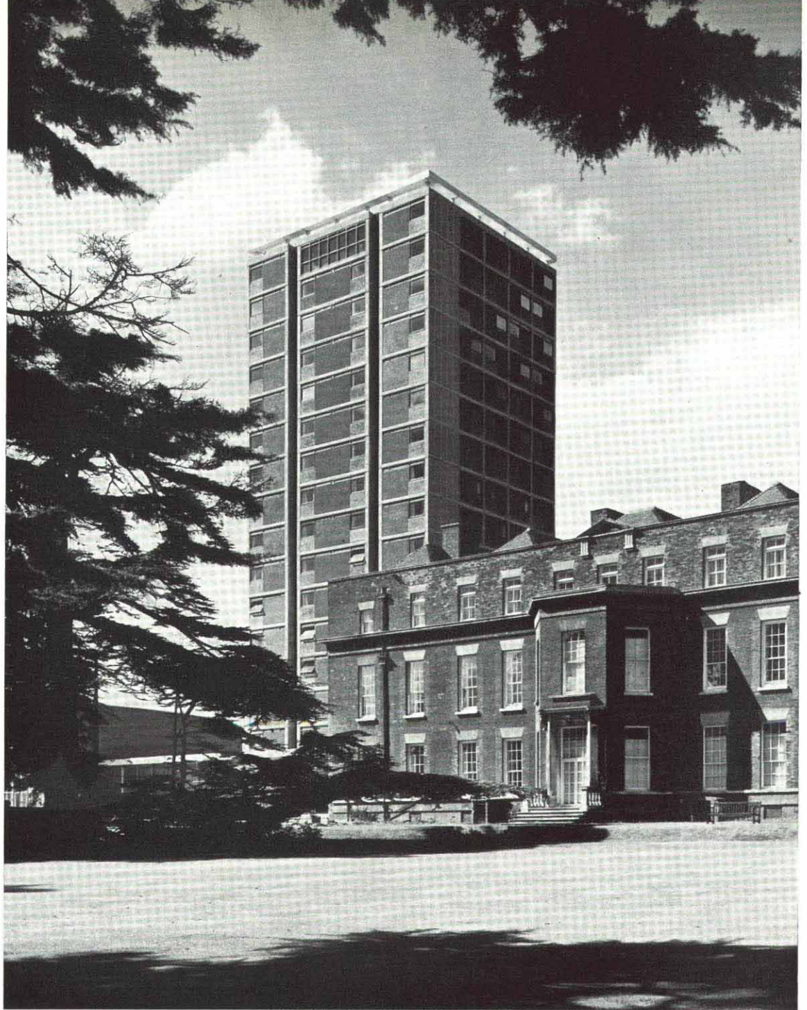
The tower block viewed from the lawns in front of the original Queen Anne mansion.
