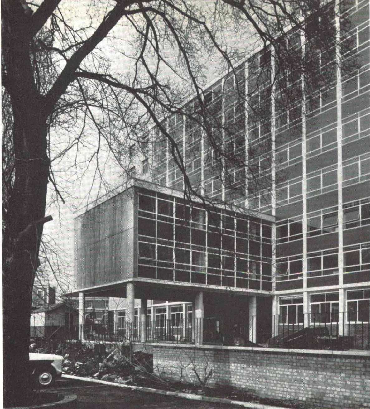
Left: The projecting wing over the entrance to Yeoman House: exposed aggregate slabs on the end wall contrast with the light blue glass spandrel panels which cover much of the building.
