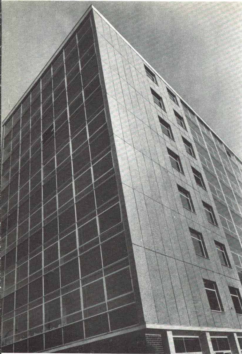
Storey-height exposed aggregate slabs provide a pleasant contrast with the curtain wall treatment on the end of the tower block.
