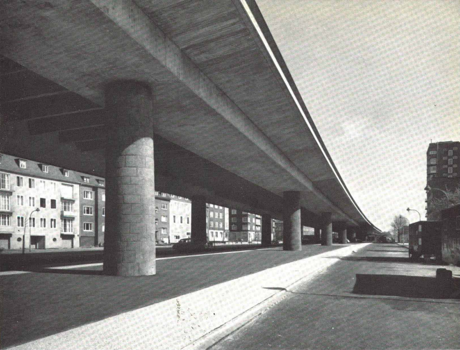
The prestressed concrete approach viaduct to the Nordbrücke on the right bank of the Rhine, the first stretch of the motorway.
