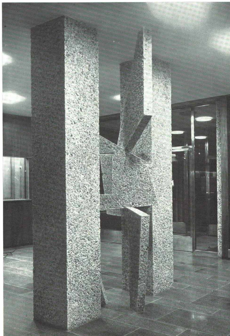
Opposite and this page: THE OFFICE BLOCK FOR THE NORWEGIAN HYDRO-ELECTRICITY ADMINISTRATION, Oslo, entirely built of Naturbetong inside and out. A stream with shallow waterfalls runs along the front. All external concrete elements are textured, including the edge beams, gable end walls and entrance canopy. Inside, the technique is dramatically carried through to such details as the concrete balustrades around circular light wells which extend one over the other above the entrance hall (far left), the relief mural in the entrance hall (above) and the sculptured column also in the hall (left). Artist: Odd Tandberg. Architects: Lykke Enger and Knut Enger.
