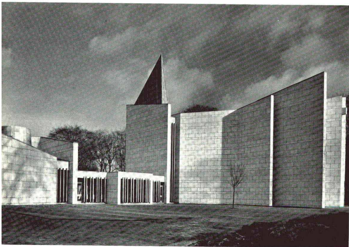
External materials are restricted to the white concrete blocks, laid in varying course heights, red cedar window frames and doors, and zinc for the covering of the triangular lantern of the Mortonhall chapel and round drum of the Pentland chapel.
