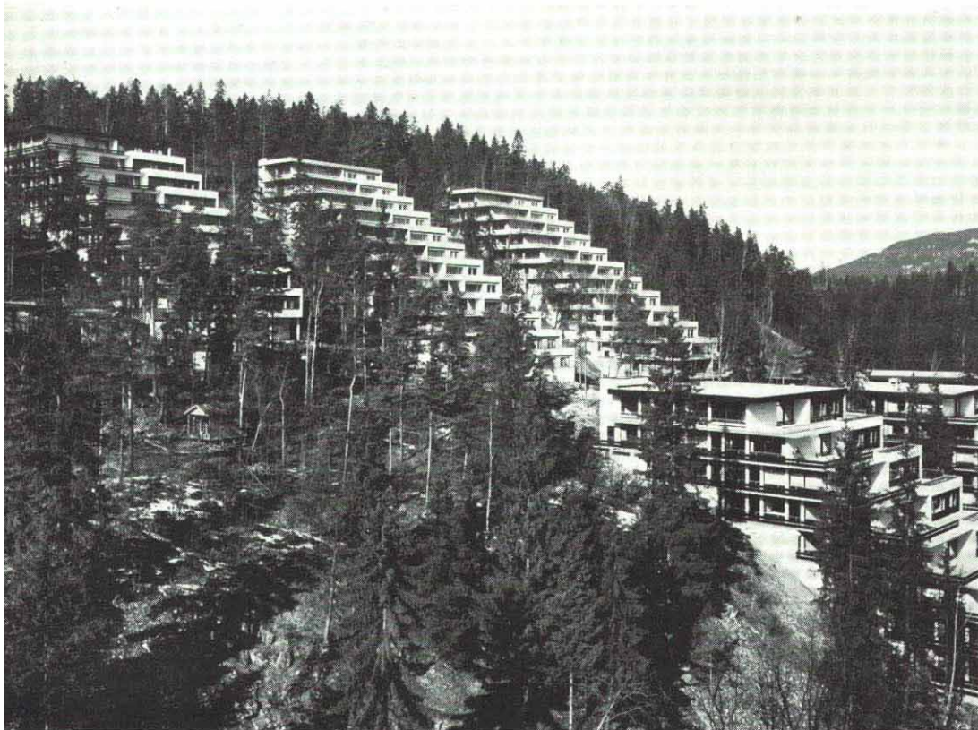
Top left and left: HOUSING AT ULLERN on the outskirts of Oslo. The flats are built into a 35° hillside and have reinforced concrete frames with timber balustrades. There are fifty-four flats in six different blocks. Architects: Olav Selvaag, Anne Tinne and Mogens Friis.
