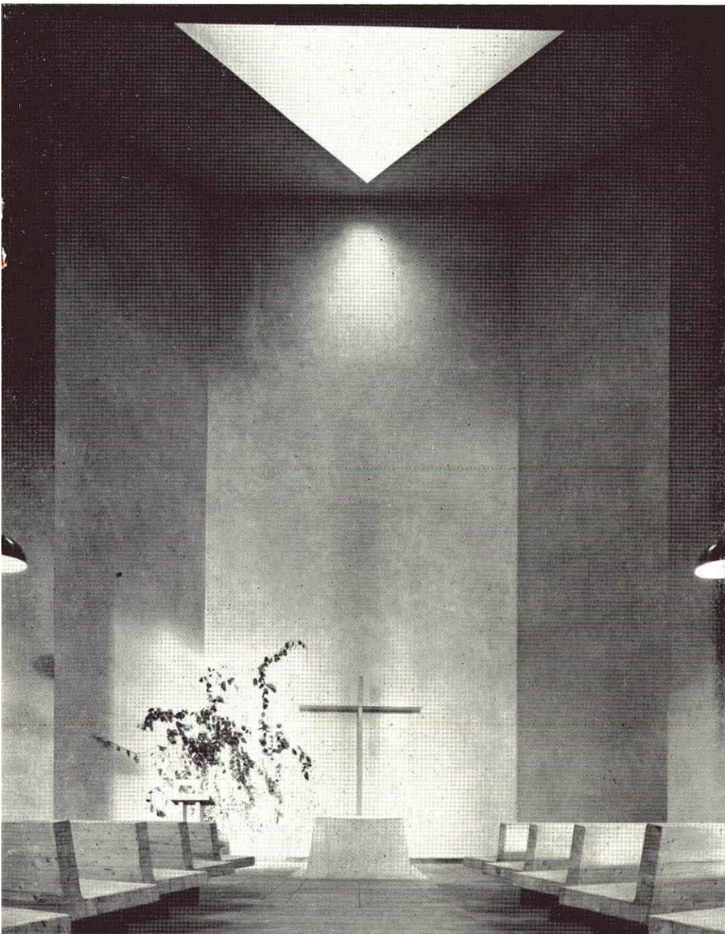
The simple and subtly-lit interior of the Mortonhall chapel. Finishes are white acoustic plaster, ceiling of natural pine, and pews of laminated pine planks on concrete blocks.
