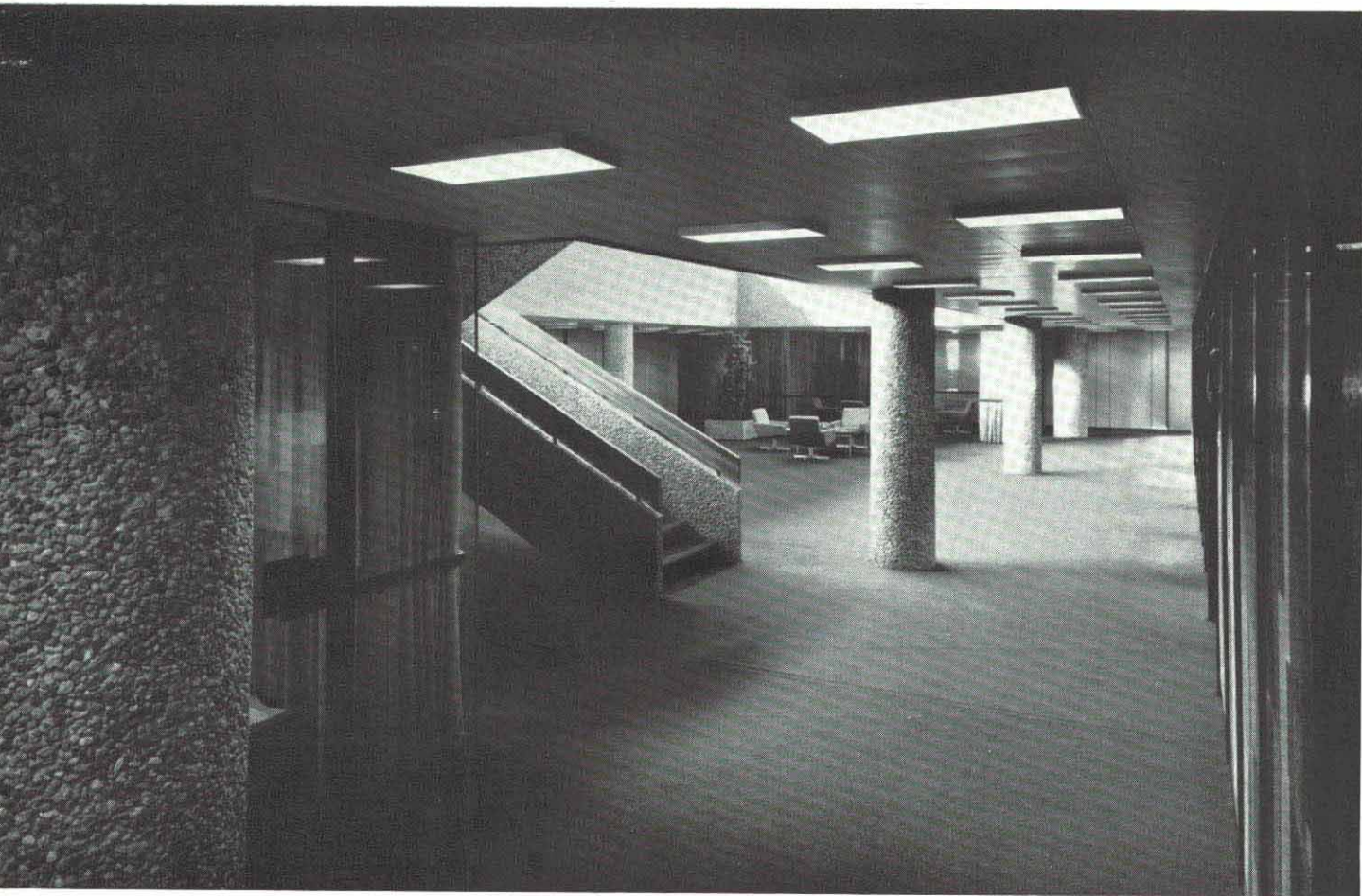
The office building for the ELECTRO-CHEMISTRY ADMINISTRATION (ELKEM) BUILDING — see also page 15. This quietly harmonious interior occurs in a reception area on the top floor. All the concrete elements are in exposed Naturbetong—columns, stair balustrades and edge beams around the gallery. The concrete effectively contrasts in texture with soft carpets and fabrics. Architect: Erling Viksjo.
