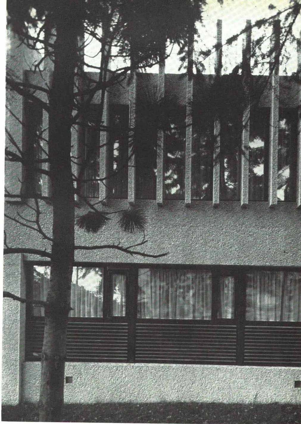
Below opposite and this page: VILLA IN ECKERSBERGSGATE, in a suburb of Oslo. It is entirely built of Naturbetong using a crushed aggregate graded from \frac{1}{2} in. to 1\frac{1}{2} in., and sandwich-construction walls. The evenly textured concrete is exposed outside and in, providing an unusual degree of unity between exterior and interior. Far left below: View from the garden showing deep-set windows and pool. Left below: Detail of roof beams. Right: The Naturbetong technique does not preclude thin elements such as these vertical fins on the upper part of the house, sandblasted on both sides. Below: Interior views of the living room and a bedroom showing the suitability of the technique for interior domestic use (see also front cover). Architect: Inge Hovig.
