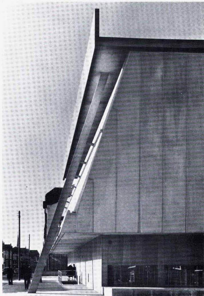
View along one of the glazed walls showing the prestressed concrete external columns.
