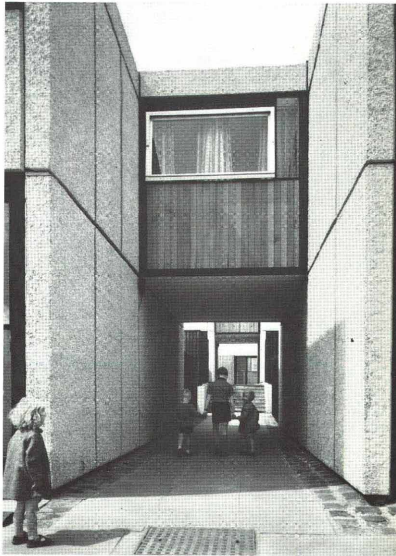
A way through between the prefabricated concrete walls faced with calcined flint.
