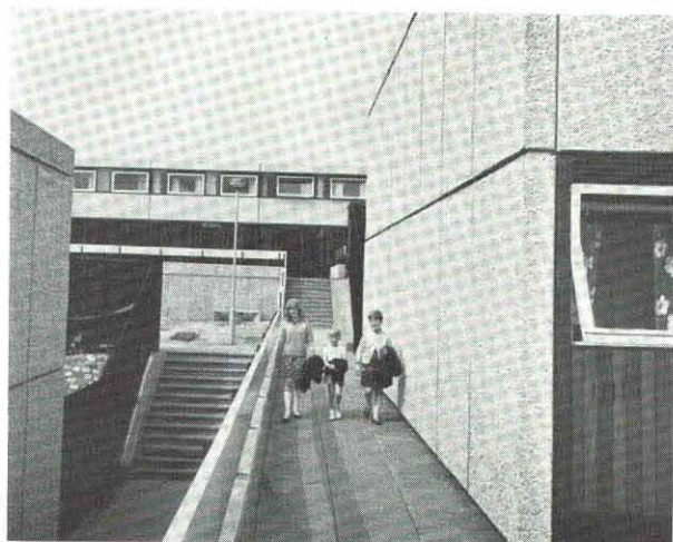
Walkway approach to flats.
