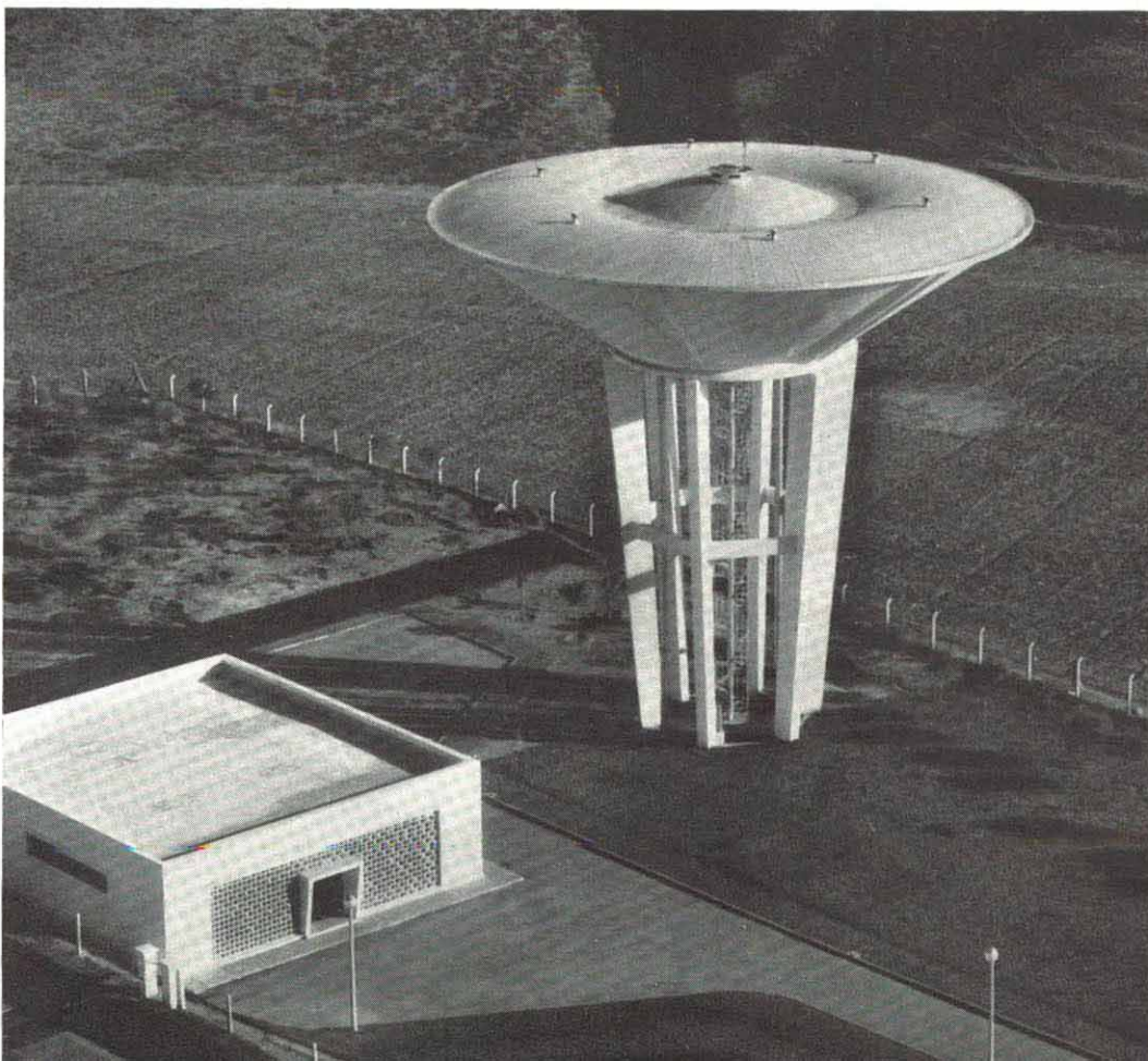
Conical, circumferentially-prestressed water tower in Rabat, Morocco.
