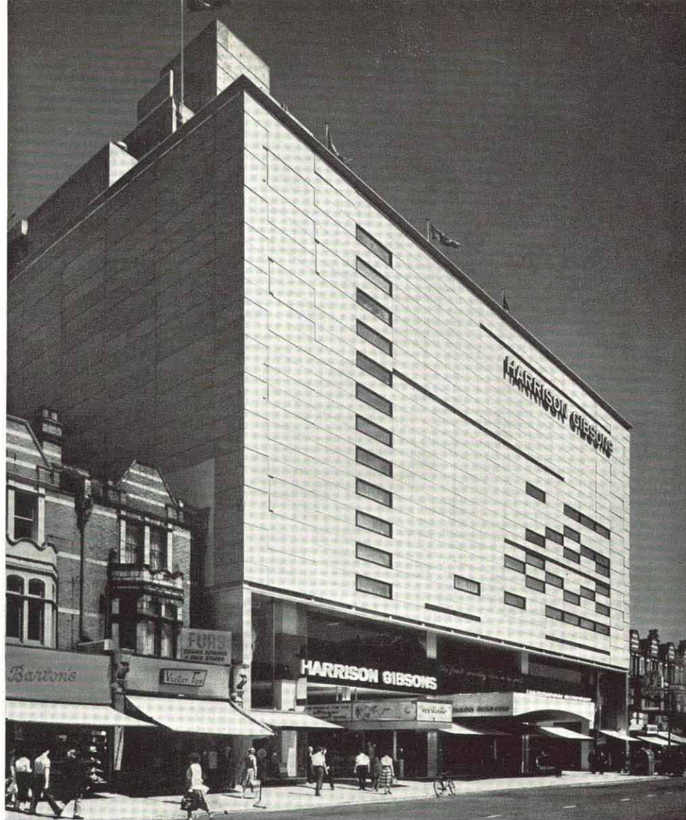
The street elevation of Harrison Gibsons: precast facing slabs and free fenestration make an unusual façade.
