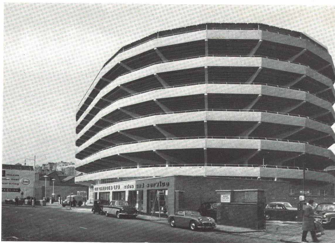
The garage from Rupert Street: the parapets are exposed-aggregate panels.
