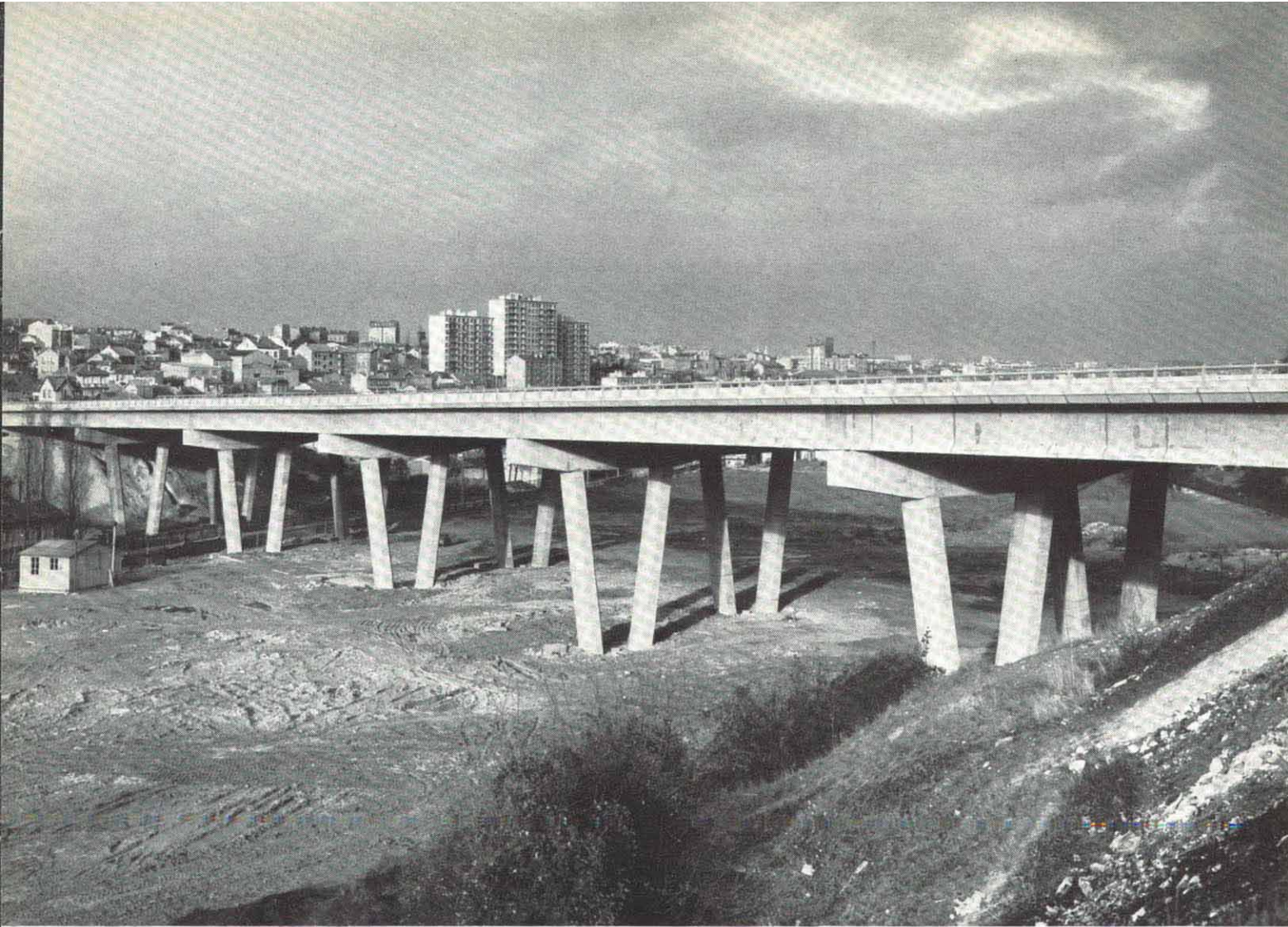
This precast prestressed viaduct carries the motorway for a distance of 730 ft. over the valley of the Bièvre at Arcueil.
